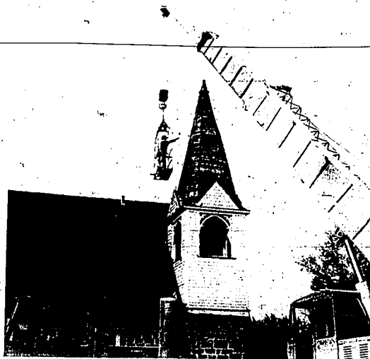
Steeple roofed THE Shoshone Methodist church got a new roof on its steeple Tuesday. The project is part of a remodeling work which has been going on at the church the past several years. Members are doing most of the work themselves.
