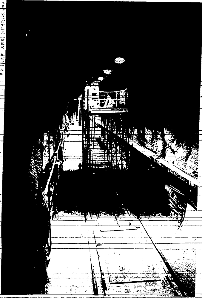
Construction scaffolding stands in tunnel carved in granite where nuclear 'trash bins' await use
