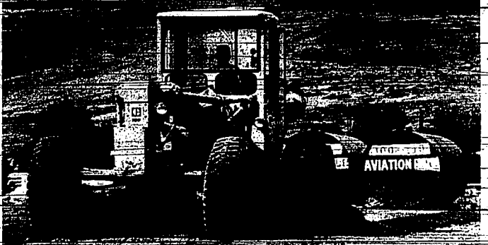
This grader is working on the new airport runway project, one of many works going on in Jackpot.
