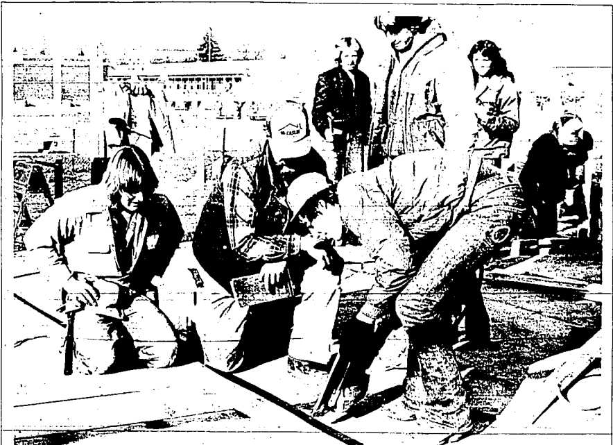
Burley senior Gib Rokich secures wall studs with a nail gun under the eye of building trades class instructor Bandy.
