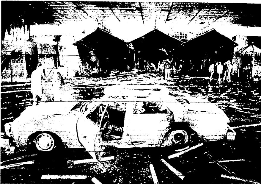
A fireball of flame totally destroyed the front area of the MGM hotel—crisping cars and melting metal
