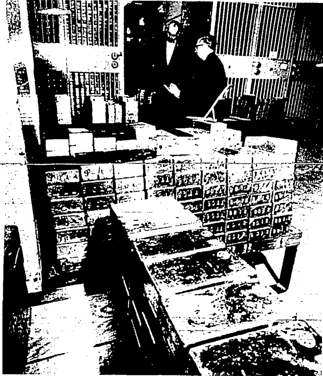
Gold destined for Iran is stacked in the Federal Reserve vault
