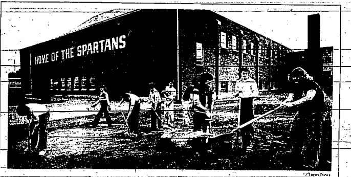
Minidoka High School students spent Monday afternoon preparing ground for landscaping.
