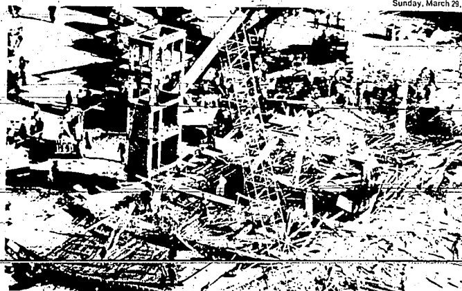
Only the central elevator shaft still stands at site where condominium collapsed Friday
