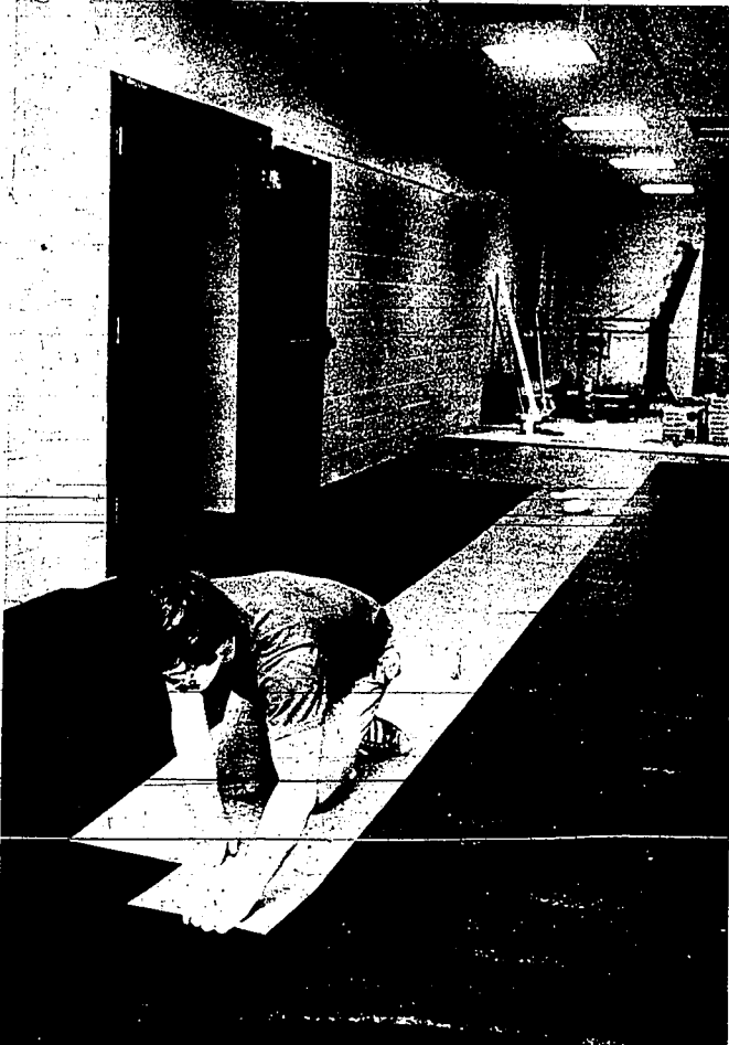
Ardell Brown of Meridian lays floor tiles in the Kimberly elementary school addition
