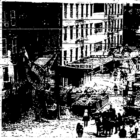
Crowd gathers in street around New York tenement which collapsed
