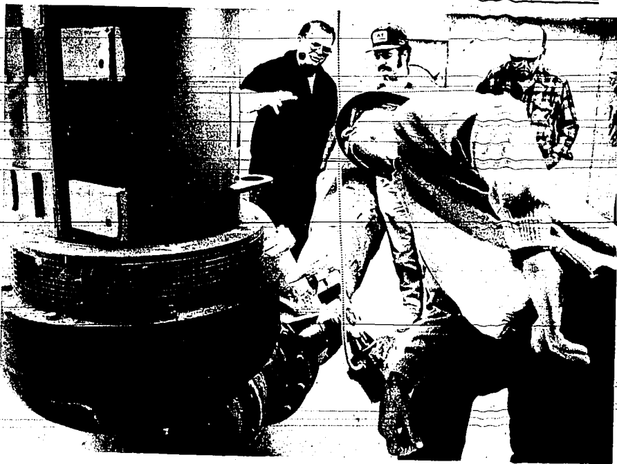
PUC member Richard High checks the details of a generator during the commission's tour of hydro power sites
