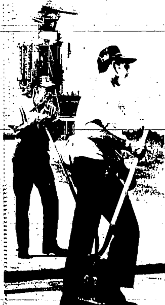
Road repairs, shuttle work both proceed
