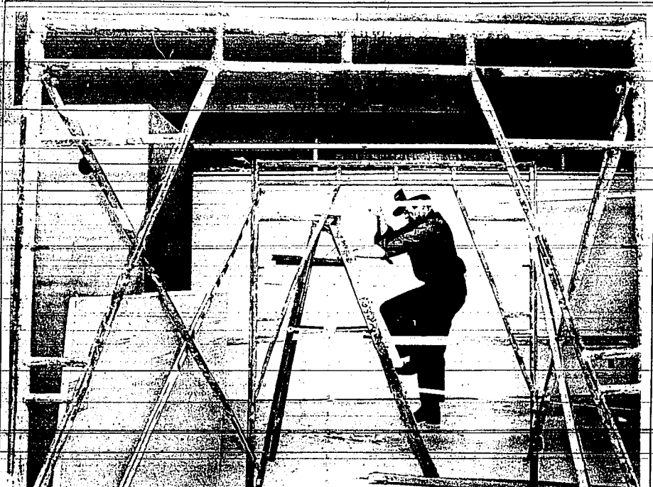
Framed in a mass of scaffolding, Navy Seabee Bob Kirk is one of many volunteers who have worked on the center
