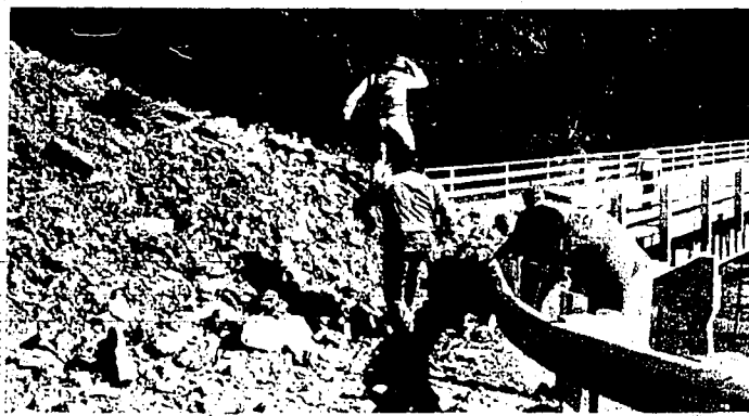
Road workers and geologists inspect landslide that blocked bridge near Morgan Hill, Calif.
