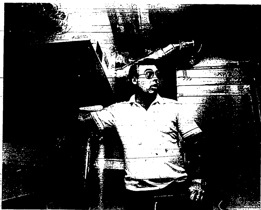
Lyle Frazier explains operation of the heat exchanger equipment, which controls air movement into and out of the house
