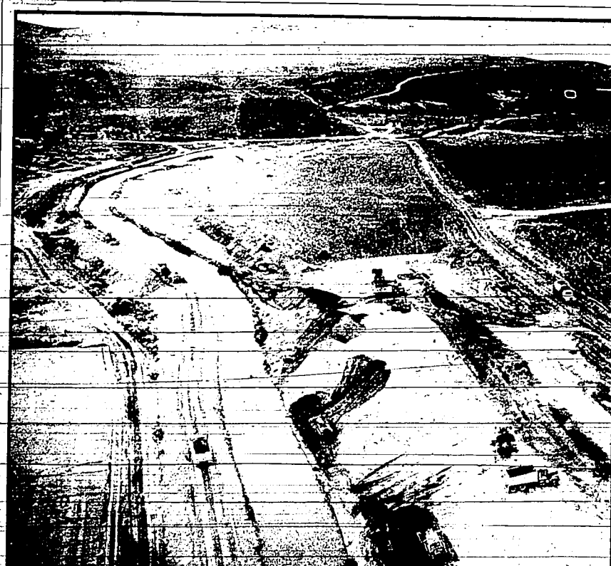
Construction crews work to enlarge an Oakley Canal Co. channel, which will divert high waters from nearby reservoir
