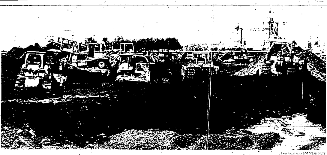
A wave of bulldozers slowly makes its way north between Oakley and Burley cutting a new channel to handle the overflow from Oakley Reservoir
