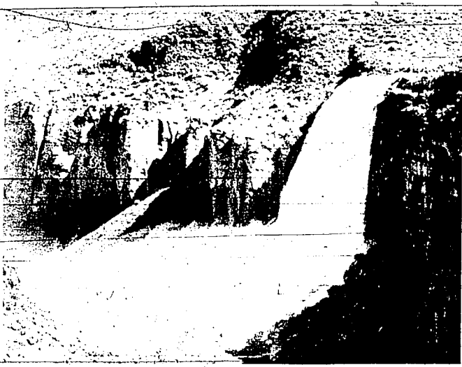
Water in Salmon Falls Creek is too high to ascertain if Walleye are moving downstream running about 1,100 cfs and I would estimate it would have to get into the 400-to-500 range before we would dare trying anything there. That was the amount they spilled in the first couple of days of testing the spillway and it appeared workable at that level. Anything above that
