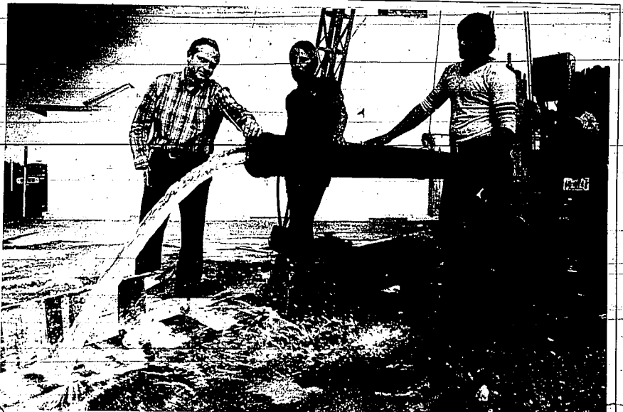
Gail Staley, left, makes a temperature check of the water being pumped from the new well behind Twin Falls High School. Times-News photo/BOB DELASO/RTT
