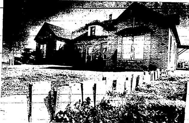
The brick exterior of Phillips' home has worn well over the past 74 years since it was built
