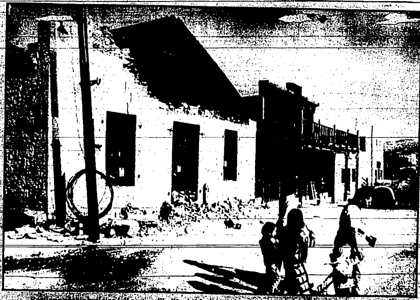
Collapsed buildings fell on two Challis children in the Oct. 28, 1983 earthquake in central Idaho.
