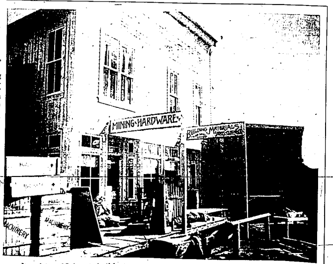
It took just 13 days to build a temporary town for filming of a new Eastwood movie
