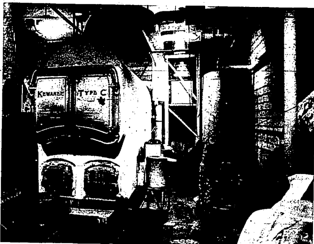
These heating pipes at Morningside Elementary School may be wrapped with asbestos
