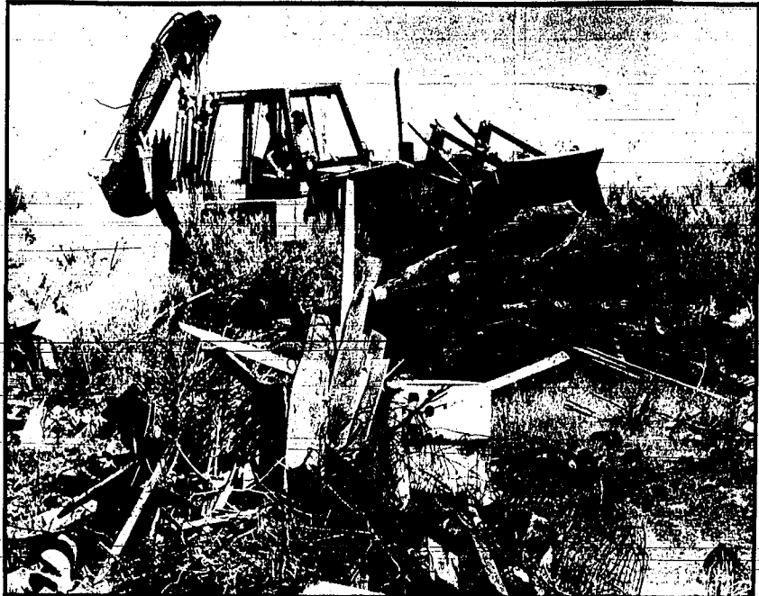
A backhoe aids in the Bureau of Land Management effort to clear trash from the Devil's Corral area
