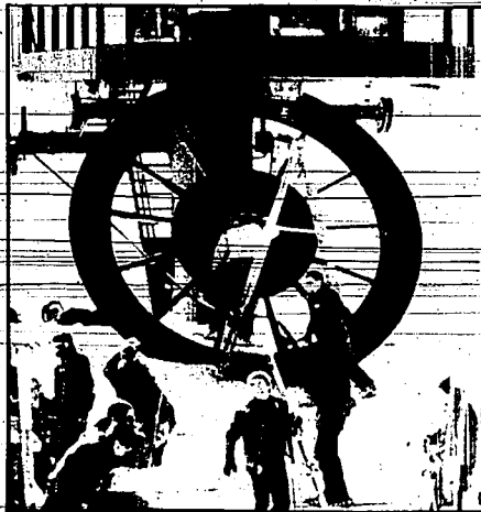
Workers inspect damage to the Keystone wheelhouse
