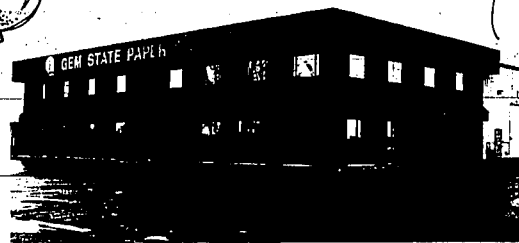
NEW LOCATION 1801 HIGHLAND AVE. EAST
