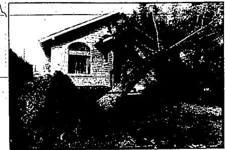
Many trees were toppled by the wind, including this pine that fell on a house on Kimberly Road
