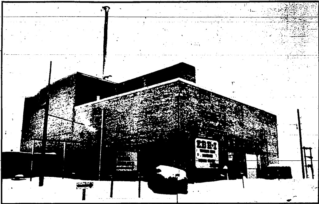
Experimental Breeder Reactor No. 1, housed in this brick building in Idaho's desert, produced first usable electricity from atomic reaction in 1951
