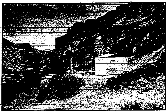
New rate levels will affect the future of small hydropower plants planned for the Magic Valley, similar to this existing plant on Salmon Falls Creek, near Buhl
