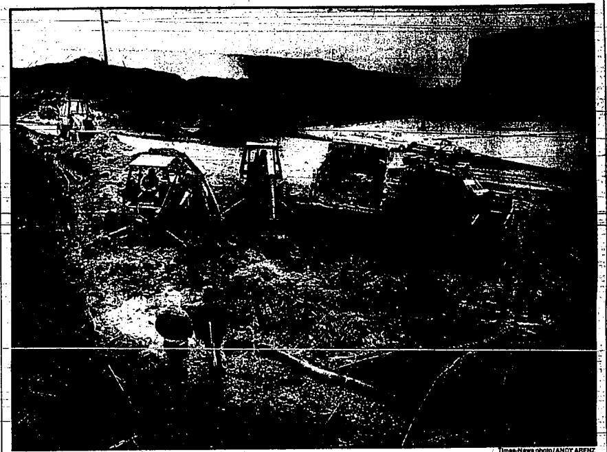
This volunteer crew, equipped with backhoes, tractors, dump trucks and shovels, builds a channel to carry spring water
