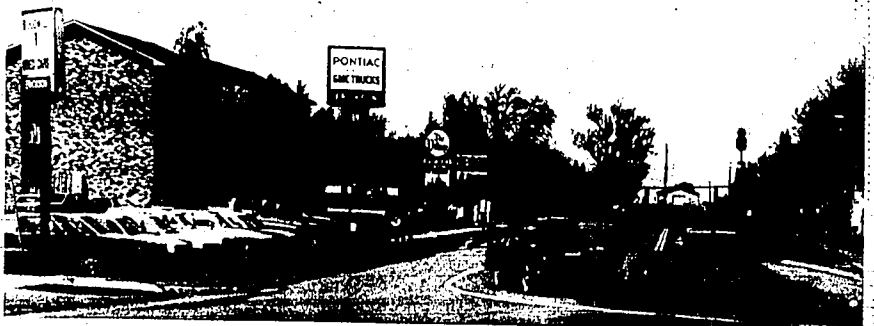
In May, 1986, this street intersection in Rexburg illustrates the rebuilding that has taken place over a decade
