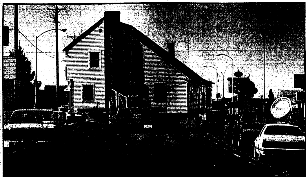
At 9 a.m. Tuesday the Warners' two-story home left its location of 30 years on Blue Lakes North, heading for a new spot near the canyon rim
