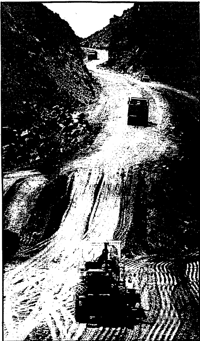
Tons of dirt are hauled down Balanced Rock Grade as the creek crossing takes shape
