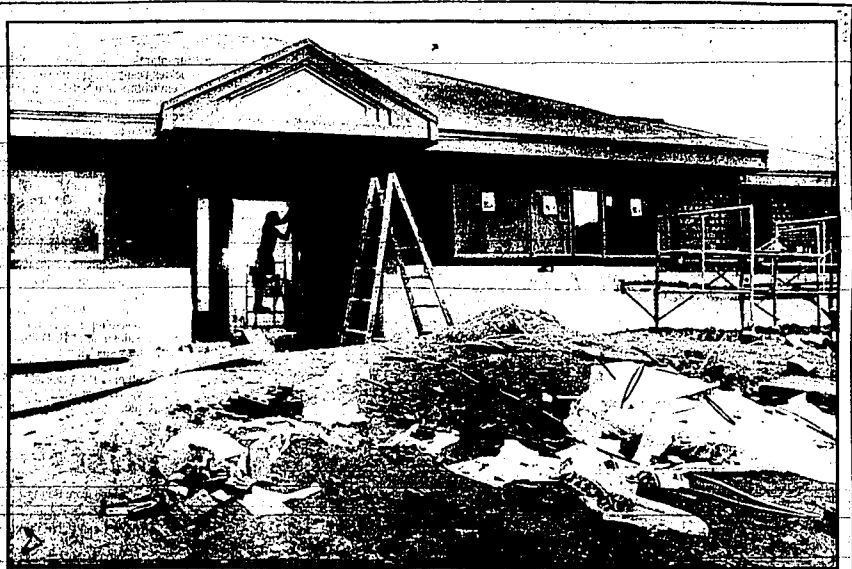
A worker installs wallpaper inside new housing facility at the State School for the Deaf and Blind at Gooding
