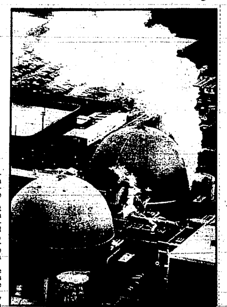
Aerial view of the Surry nuclear power plant after a steam pipe in the turbine ruptured
