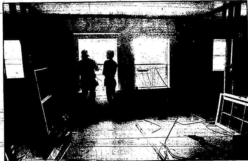
Two workers replace the first of 180 wooden windows in one of the 36 units of the 66-year-old apartment building
