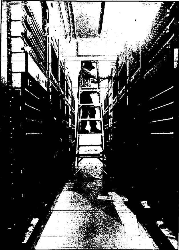
Dan Kleinsmith levels the bays which hold the all-electronic switching equipment
