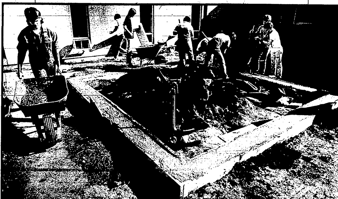
Members of Norm Redd's building and construction class lay the cement foundation of the new greenhouse at Robert Stuart Junior High School.
