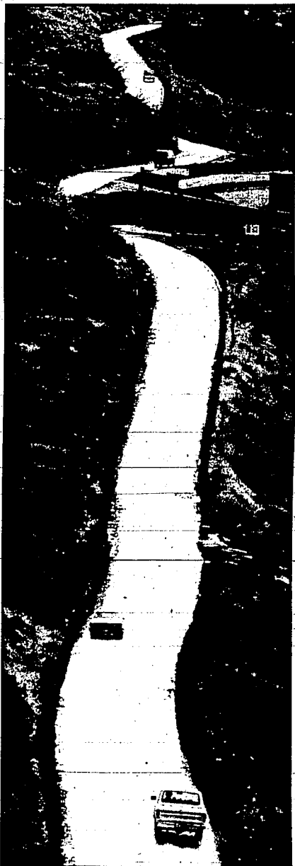
A view of the aging Clear Lakes Grade, looking east
