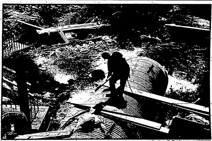
Workmen construct a wall with gate below Niagara Springs. The wall will be used to divert water for fish operations.
