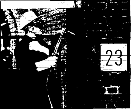
Wrecking worker detaches the prison's main gate
