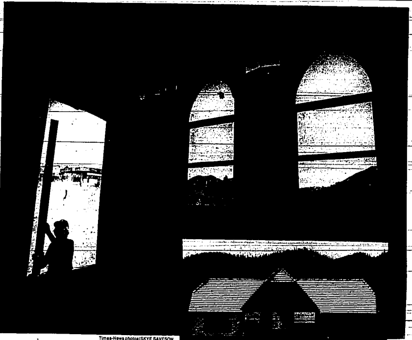
Ted McConville measures a facing board for a doorway while working on his replica of the Dollarhide house.
