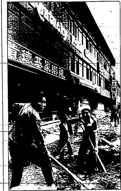
Colonel goes to China Chinese workers prepare the street in front of Beijing's soon-to-open Kentucky Fried Chicken restaurant, believed to be the first American-style fast food franchise eaten in China. Construction delays have set back the scheduled Sept. 29 opening by several weeks.
