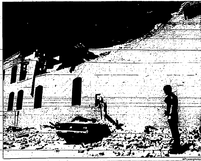
Bricks from this collapsing wall in Whittier, Calif., crushed a parked Mustang
