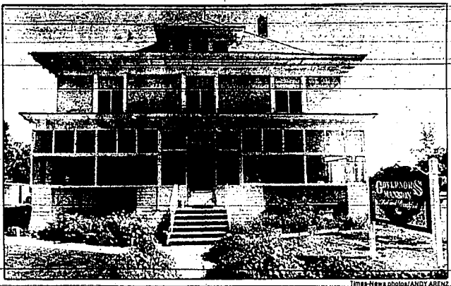
This colonial revival mansion was reborn as Shoshone's first bed and breakfast inn
