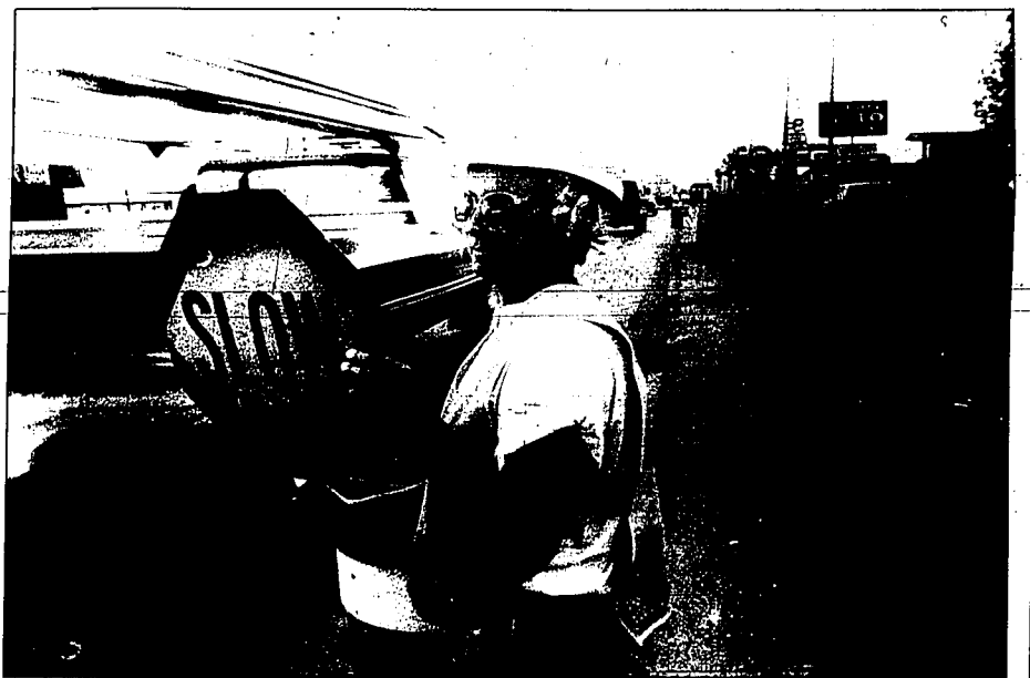
Karen Wright, Kimberly, signals to Blue Lakes Boulevard traffic. The widening project should be finished within three weeks.
