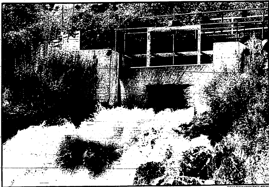
Natural rock facing will be added, the walkway removed and head gates renovated at the Niagara Springs diversion
