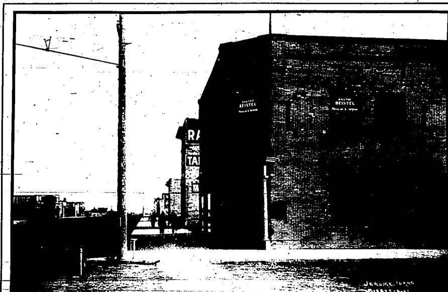
The First National Bank building and downtown Jerome as they were early in the century (above), and today (below)
