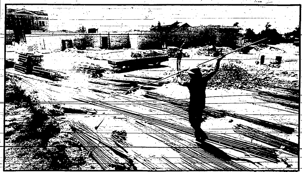
Men at work Worker Jeff Mathis lifts a steel bar during construction of the new Twin Falls County Jail. After three months of work, the facility, located near the courthouse, is taking form. County commissioner Jim Fraley said the project, expected to be completed by spring, is on schedule.
