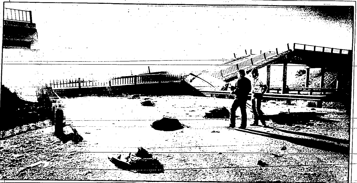
Amid bags of peat moss, truckers Ken More, left, and Dave Perkins, both of whom narrowly escaped injuries, look over collapsed bridge on I-84
