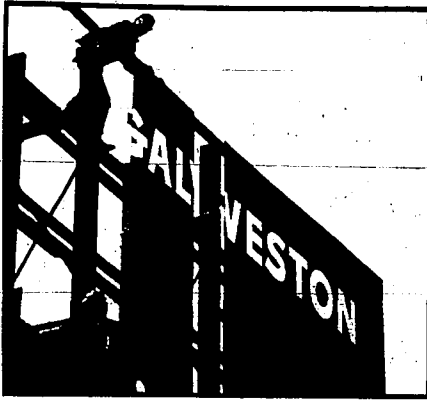
Crew removes sign panels as Galveston, Texas, gets ready
