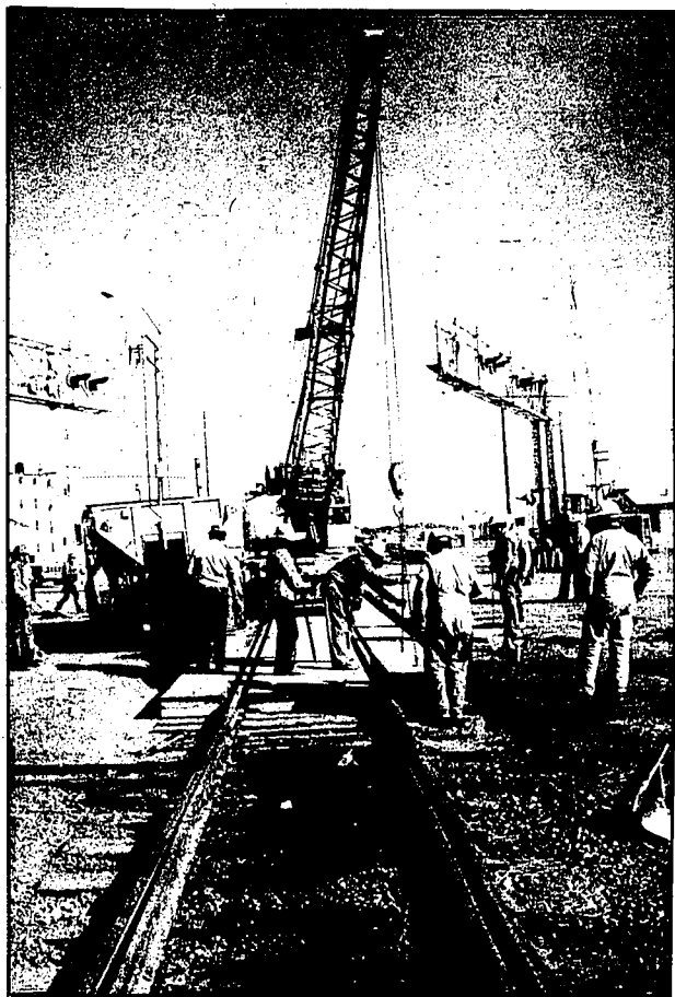
State and Union Pacific workers install concrete railroad crossing on Shoshone Street
